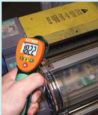
Electrical Troubleshooting for hot spot detection
